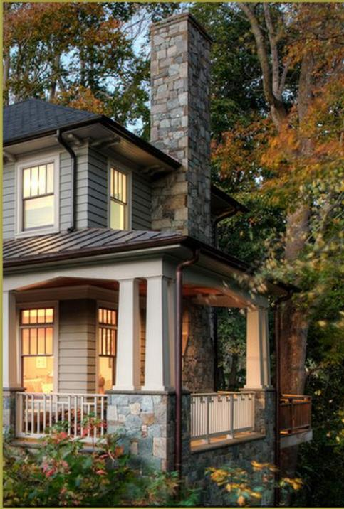
Windows may not be set in chimneys, even if the flue can be fitted beside them, because this would appear structurally unsound. Nor should windows be located under them because the chimneys must extend to the ground. Similarly, windows may not be placed over the vent of direct-vent fireplaces. Stone or brick is the preferred cladding for chimneys but stucco is also acceptable with good detailing.
